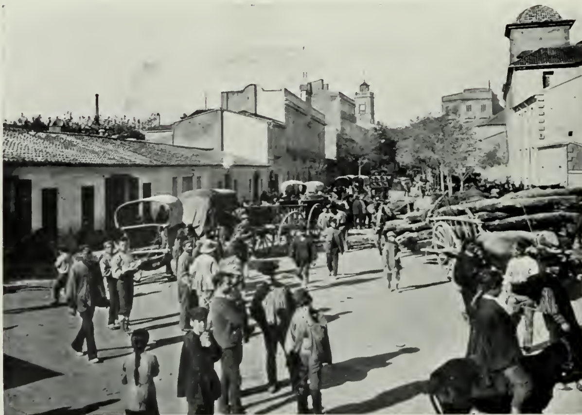
ENTRANCE TO THE TOWN BY THE PUERTA DE SANTA LUCIA
